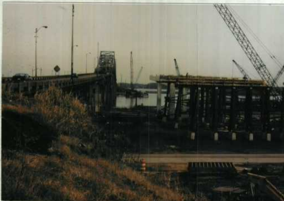
Work started on the Tennessee River Bridge at Decatur. About six acres of refuge were lost in this construction.
