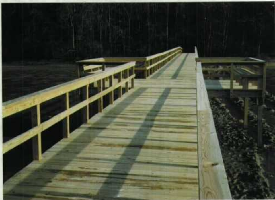
The final product was a well-constructed boardwalk at a considerable savings to the Service.
