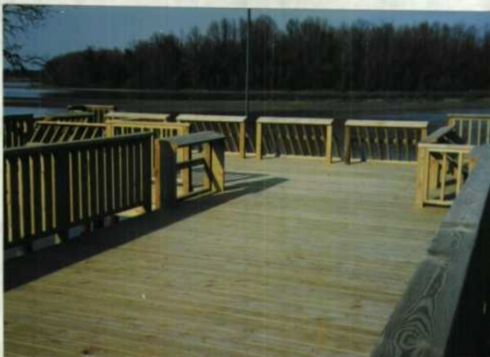
After the contractor completed the decking, refuge personnel built the rails and fishing stations.
