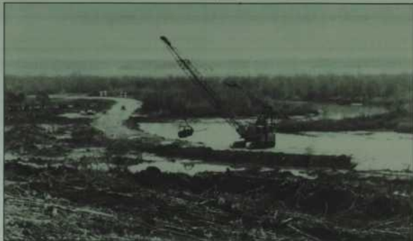
Olin cleanup workers dredge a stream channel in Lower Reach A of the Huntsville Spring Branch. This new 1,600 foot channel connects the upper and lower portions of the river area, by-passing 71 tons of DDT-contaminated sediments.
