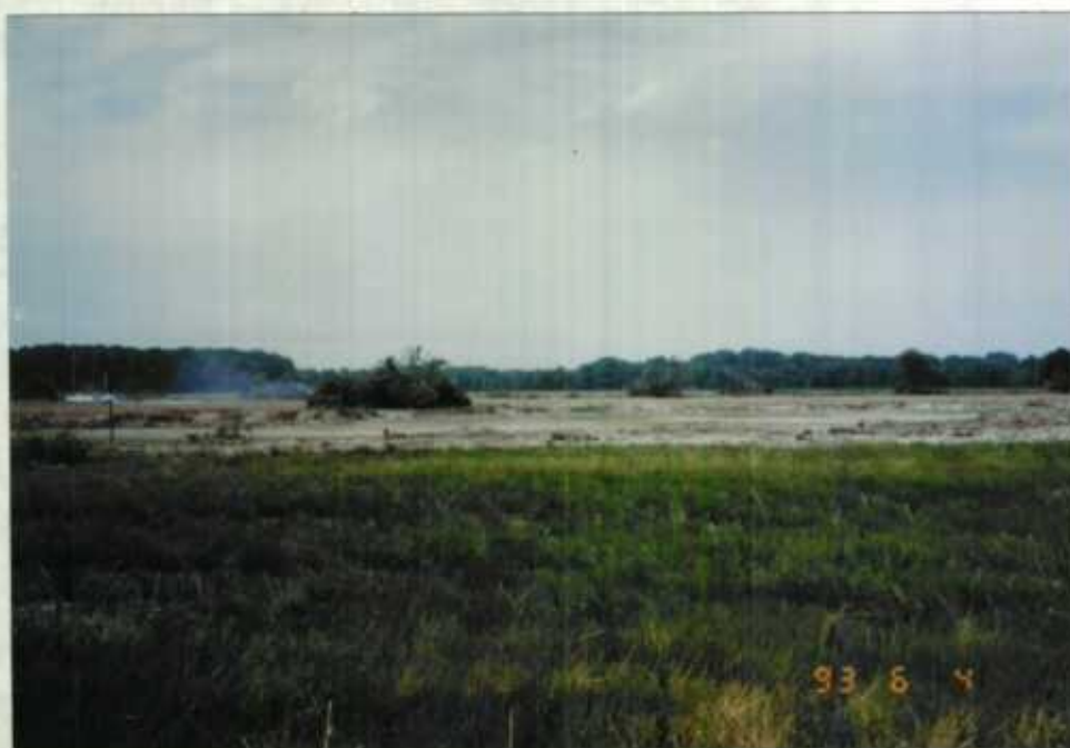
Shoreline clearing was also completed around the perimeter of the Penney Bottoms Impoundment.
