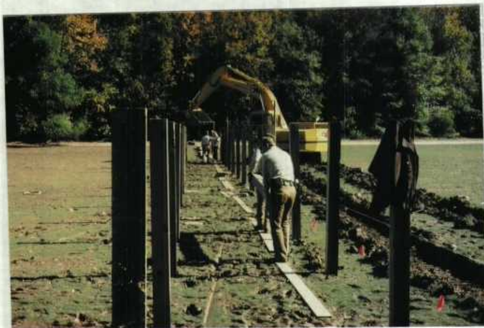
The refuge crew placed the boardwalk pilings using an excavator.
