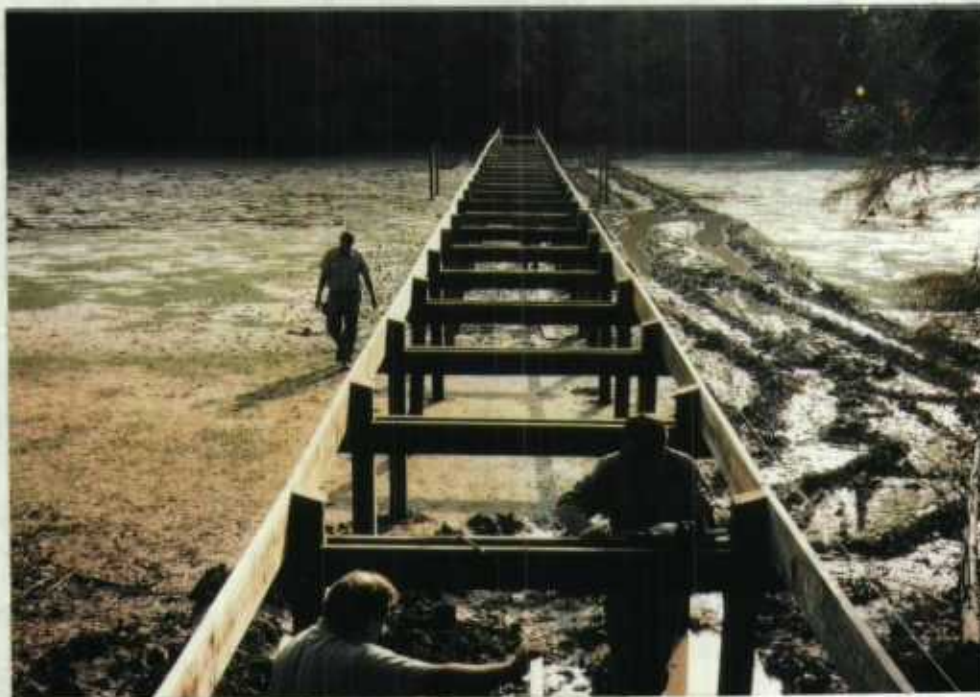
The next step was bracing the 6x6 posts and adding runners between the pairs of posts.
