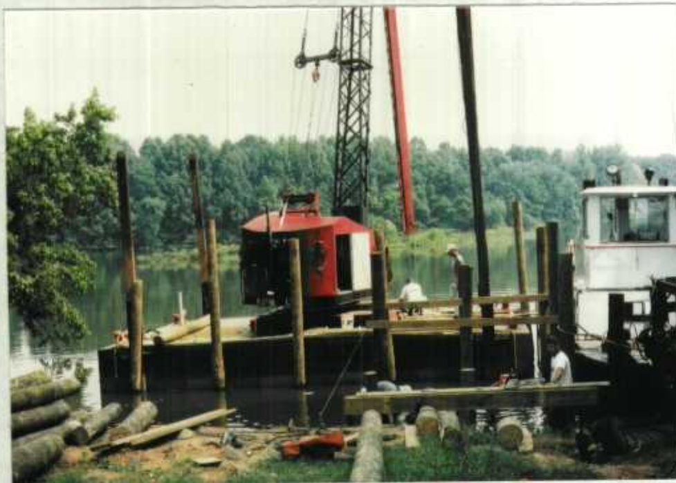
Work started on the handicap-accessible fishing pier with a local contractor driving pilings.
