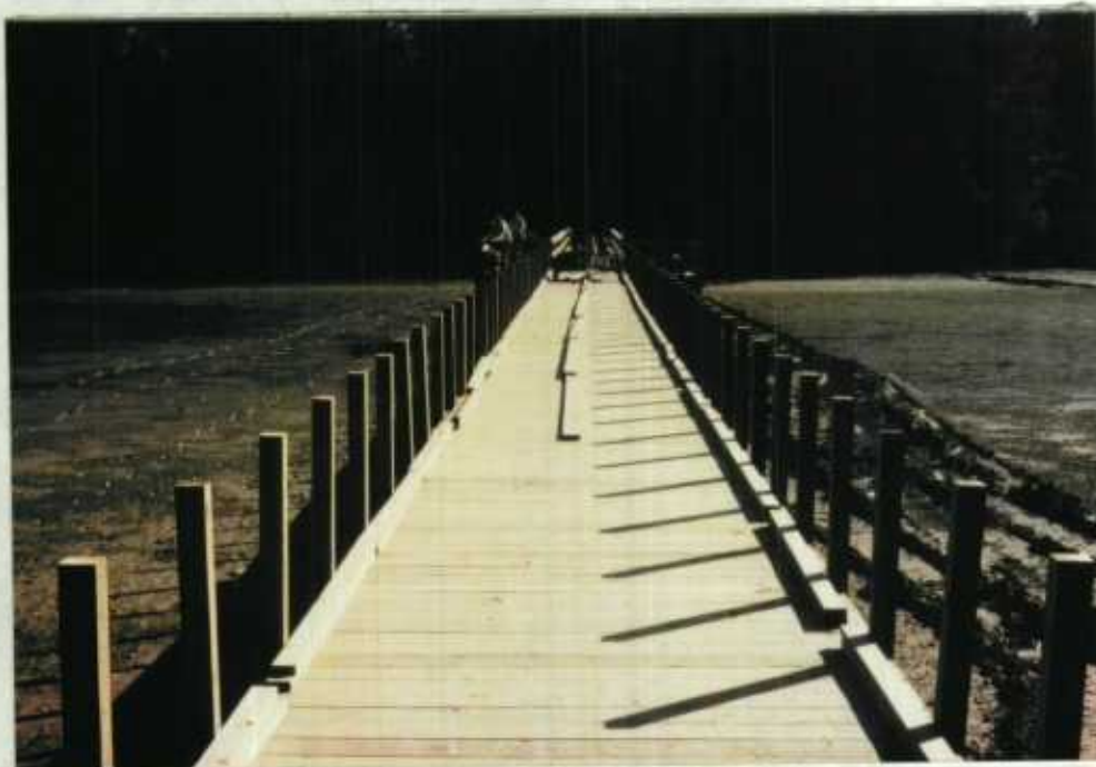
The decking and handrail posts were completed by the end of November.
