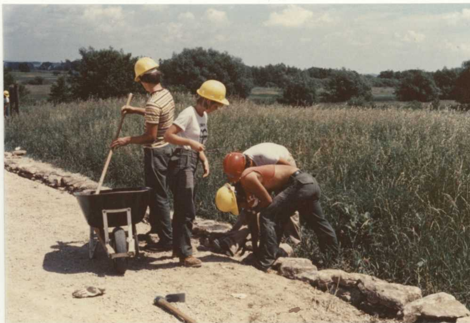
Rock was painstakingly laid to construct a 2\frac{1}{2} ft. wide wall, mortaring between all layers of rock. 7/78, Thompson
