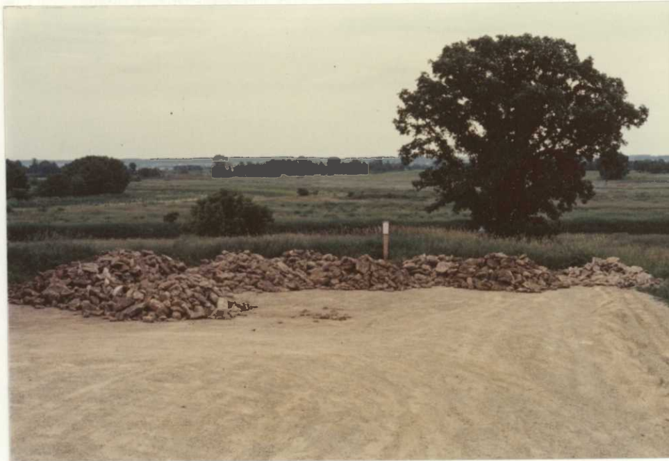
Limestone rock was gathered by YCC'ers and hauled to Peachey Rd. parking area, to be used in constructing a rock wall. 7/78, Thompson
