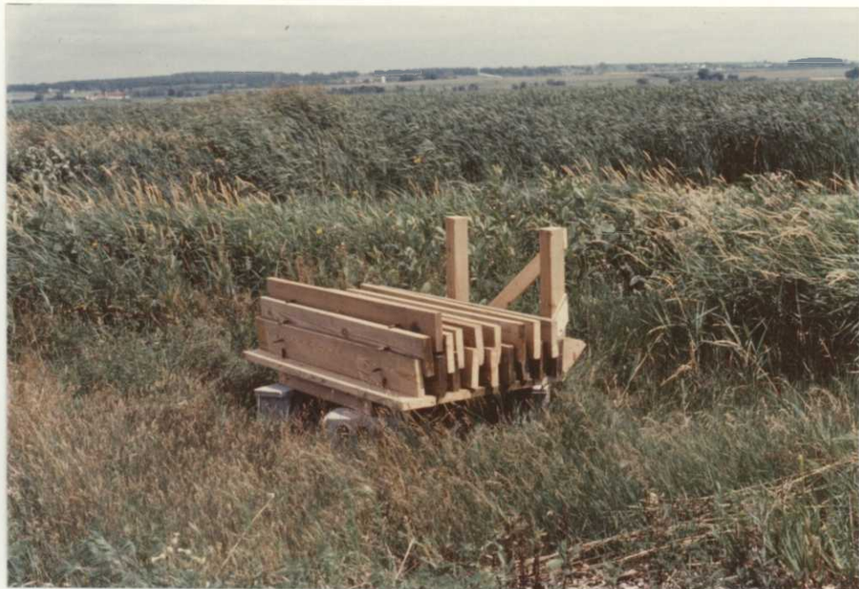
Five stoplog storage racks and stoplogs were constructed by YCC. 7/78, Thompson
