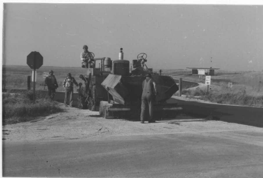
Blacktop machine working on road to comfort station. Roll 8-78, Exp. 8. Drieslein
