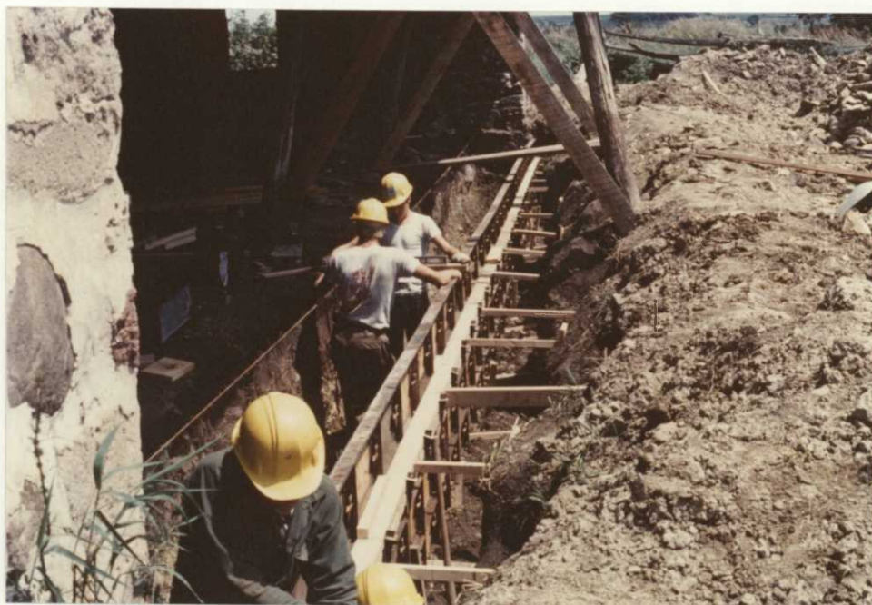
YCC'ers place cement forms in a 4-foot trench they dug in preparation for the foundation to be poured. 7/78, Thompson
