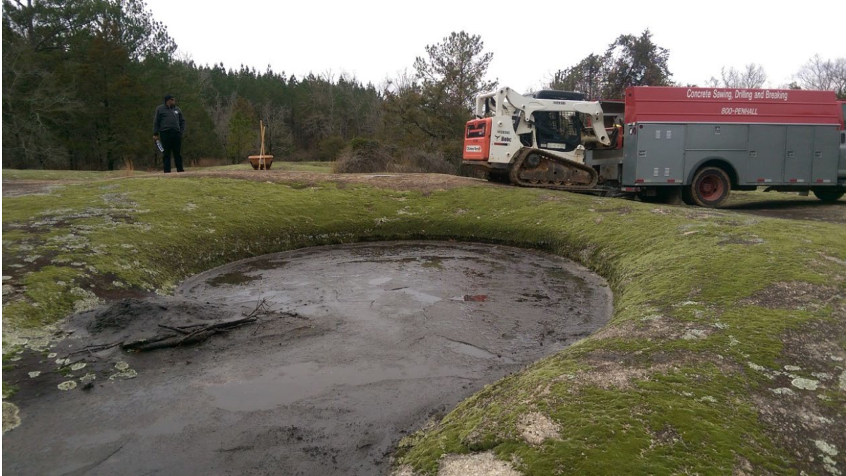
Figure 16. “Penhall contractors prep equipment for cutting. Surface water and soil were removed from the pool prior to cutting. Original soil was then replaced into the deepened pool” (Richards, 2015).
