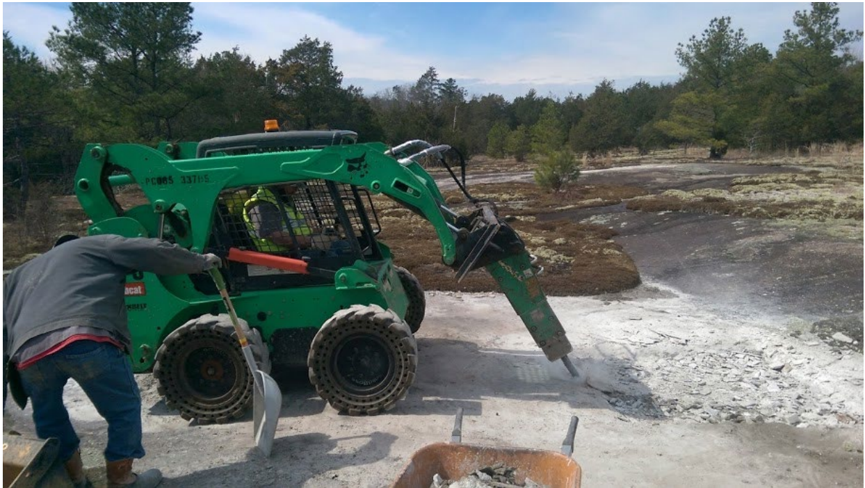
Figure 23. Excavation of overburden in Pool #3 at Heggie's Rock. Overburden was removed by wheelbarrow from the outcrop (Richards, 2016).
