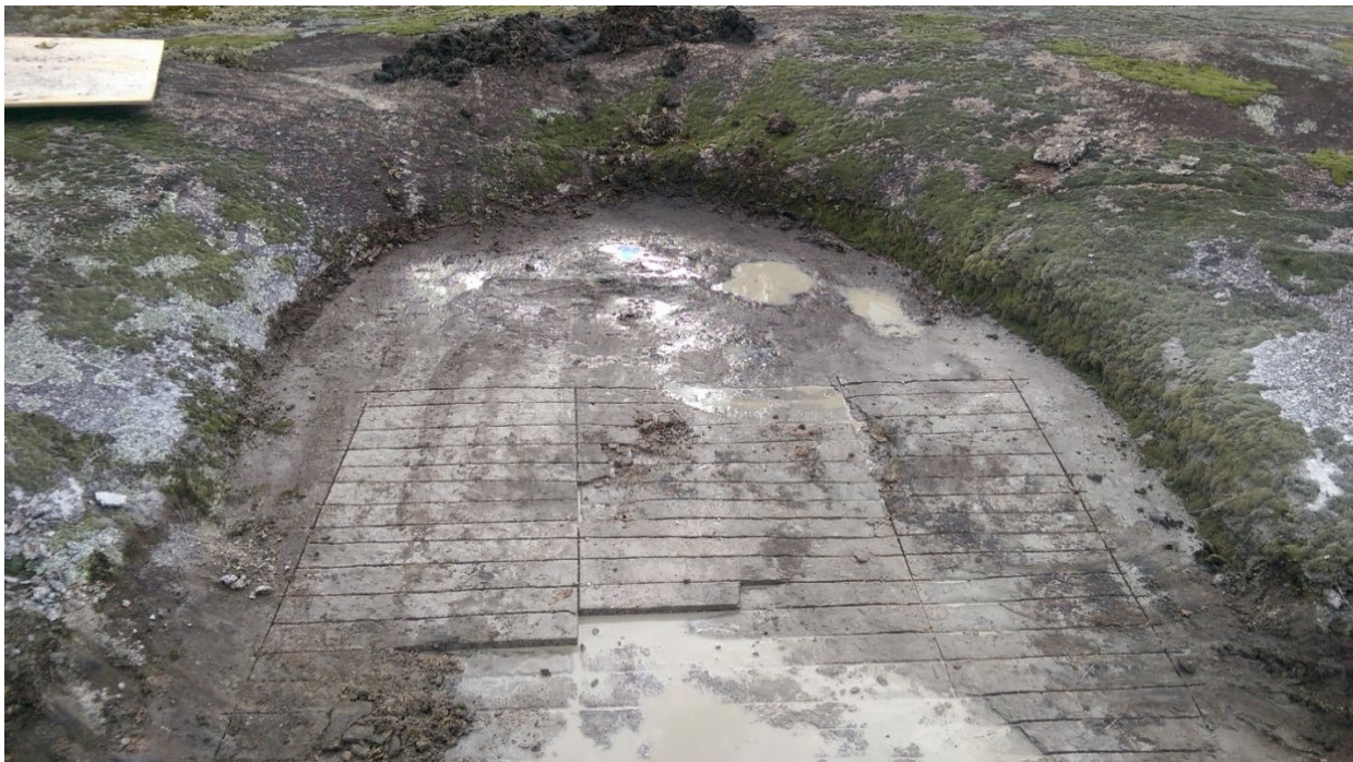
Figure 17. “Pool 2 cut to a 4” depth in crosshatched pattern. Soils excavated from the pool prior to cutting can be seen at the top of the image” (Richards, 2015). This method was used for all pools cut with a diamond blade saw. Note that here an existing depression is being deepened, not a bare rock de novo pool creation.
