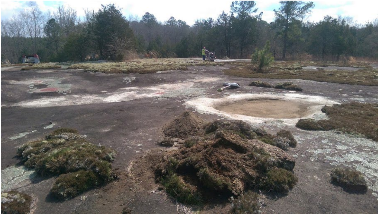
Figure 22. Penhall contractors use a diamond blade wet concrete saw to create cuts in the pools. Notice the truck in the staging area (top left) and the mats of mosses and Selaginella in the foreground. These mats of vegetation would be utilized to heal-in disturbed areas where the skid steer accessed the outcrop (Richards, 2016).
