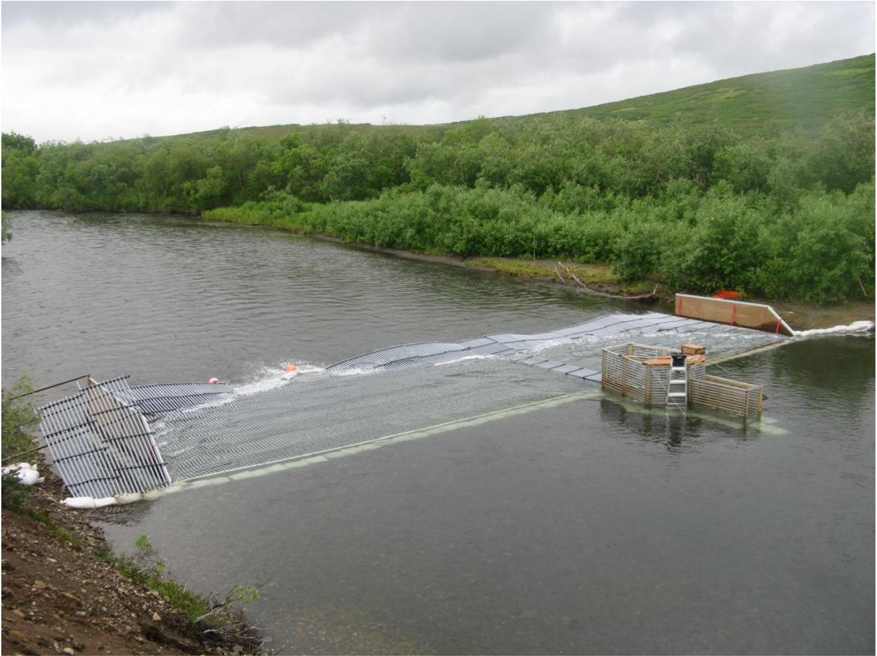
**Figure 2.** A resistor-board weir installed in Gechiak Creek, 2010. A remote telemetry station was co-located on top of the bluff .
