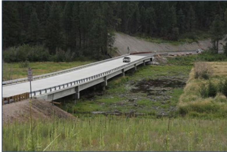
Figure 38. Construction of a new bridge on Highway 126, Jemez Mountains, New Mexico, in 2005 (photo courtesy of J.N. Stuart).
