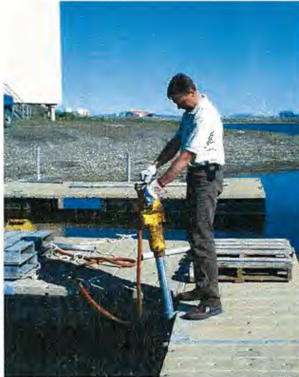
ARM Jimmy Fox works on the float plane dock at the refuge hangar in Kotzebue.
