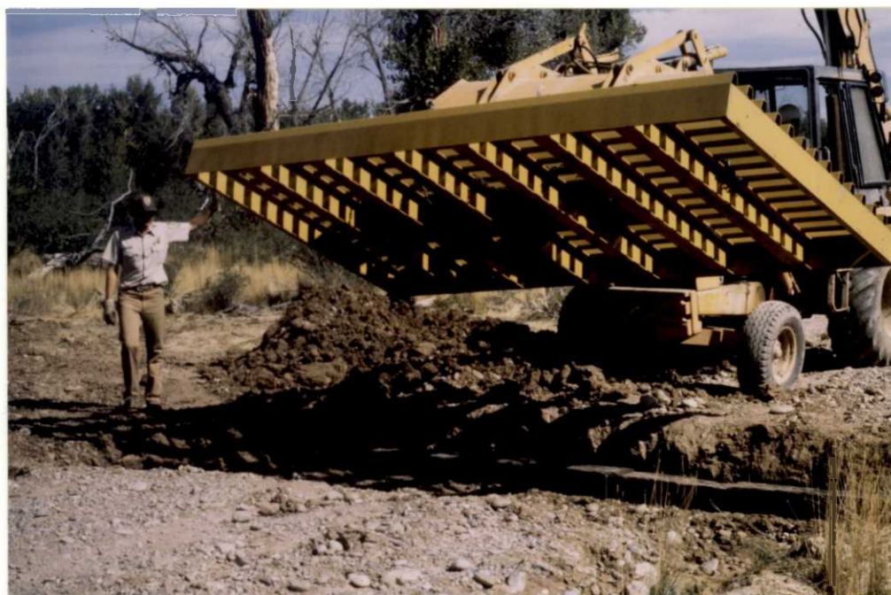
A new cattleguard being placed in the Wyasket Bottom after the original was stolen.
