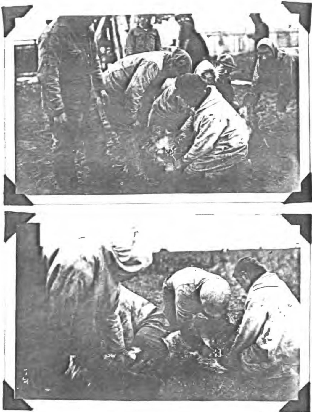
Use of Burdizzo pincers in castration of reindeer-caribou cross males Nunivak Island 1930. Upper - Placing the instrument preparatory to closing. Lower - Completion of operation.
